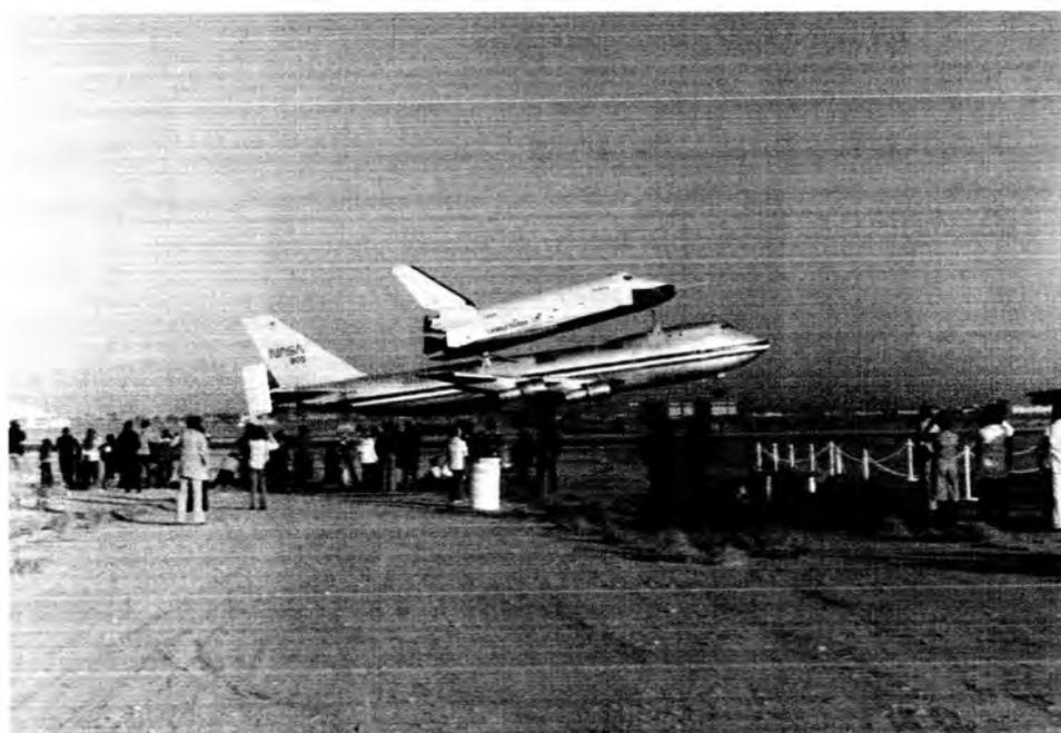
Fig. 4. The Enterprise mated to the SCA lifting off for the fifth ALT flight. (ECN 8905)
