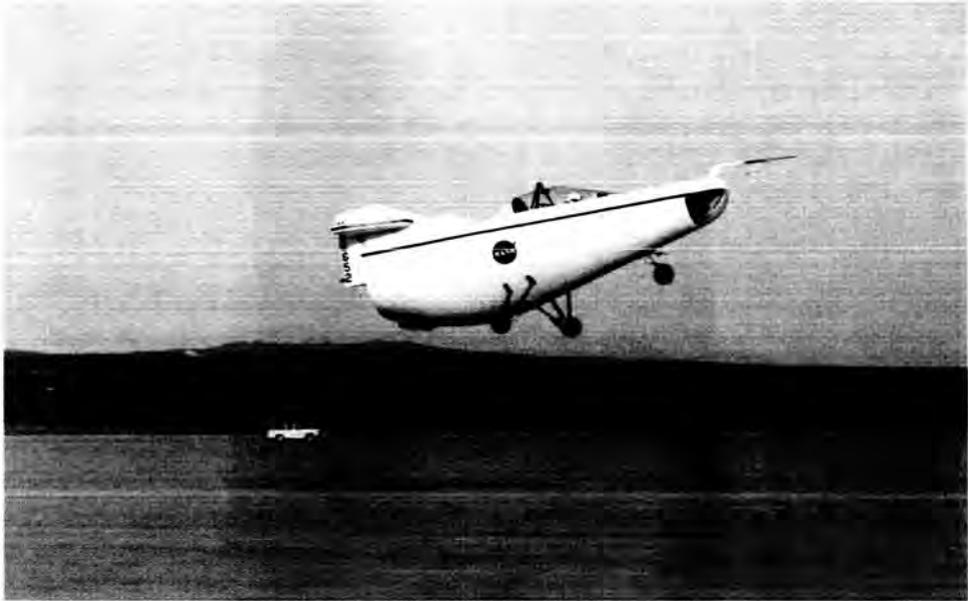
Fig. 2. A photo of the M2-F1 taken immediately after the first release from a car tow, capturing the moment of the very first free flight of a lifting body. Milt Thompson flew the M2-F1 on April 23, 1963. (E 9829)
