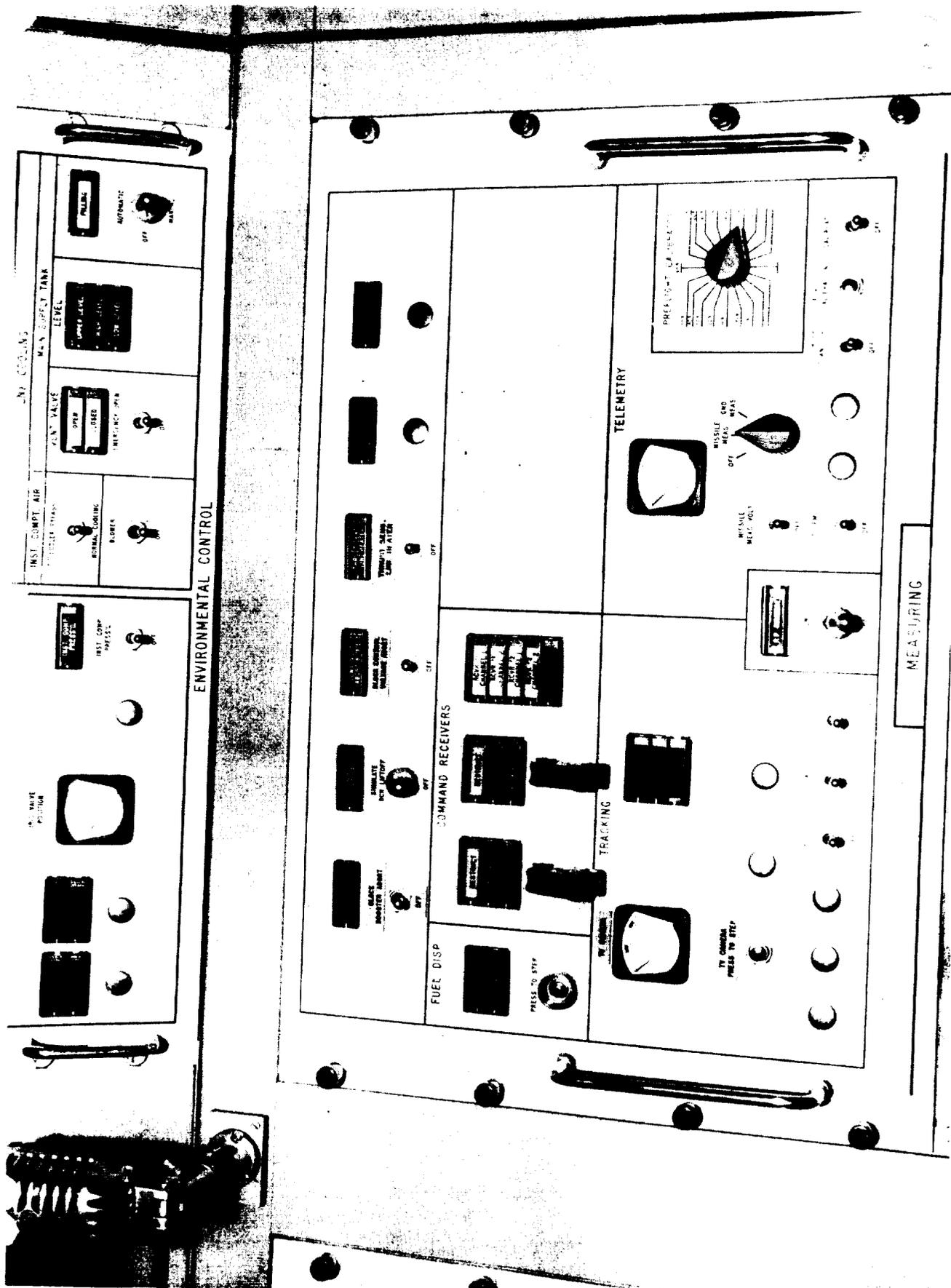
Figure 7-13. Environmental Control Panel and Measuring Panel, Blockhouse 56
