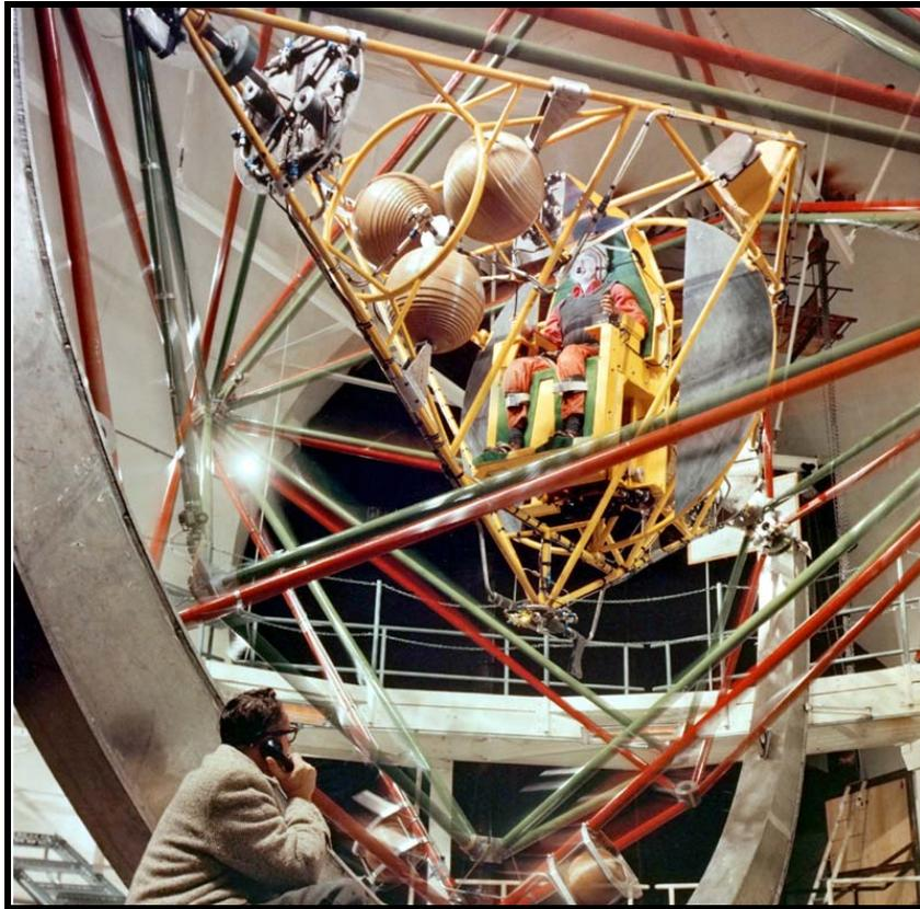
One of the problems facing man when he first begins to travel in space is whether or not he can properly orientate and control the flight of his space vehicle. The National Aeronautics and Space Administration has constructed a multi-axis test facility at its Lewis Research Center in Cleveland.
